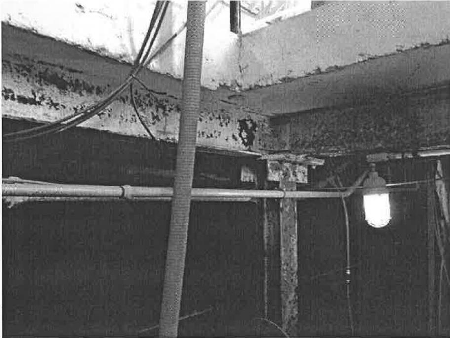
**Photo 5** View of Lead-Based White Paint (0.73-1.1%wt) on Horizontal Structural Beam near Filter#25.
