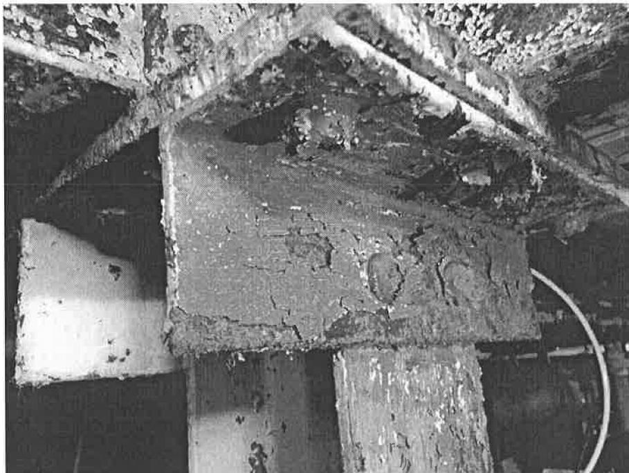
**Photo 4** View of Lead-Based Brown Paint (4.4%wt) on Vertical Structural Beam near Filter #9.
